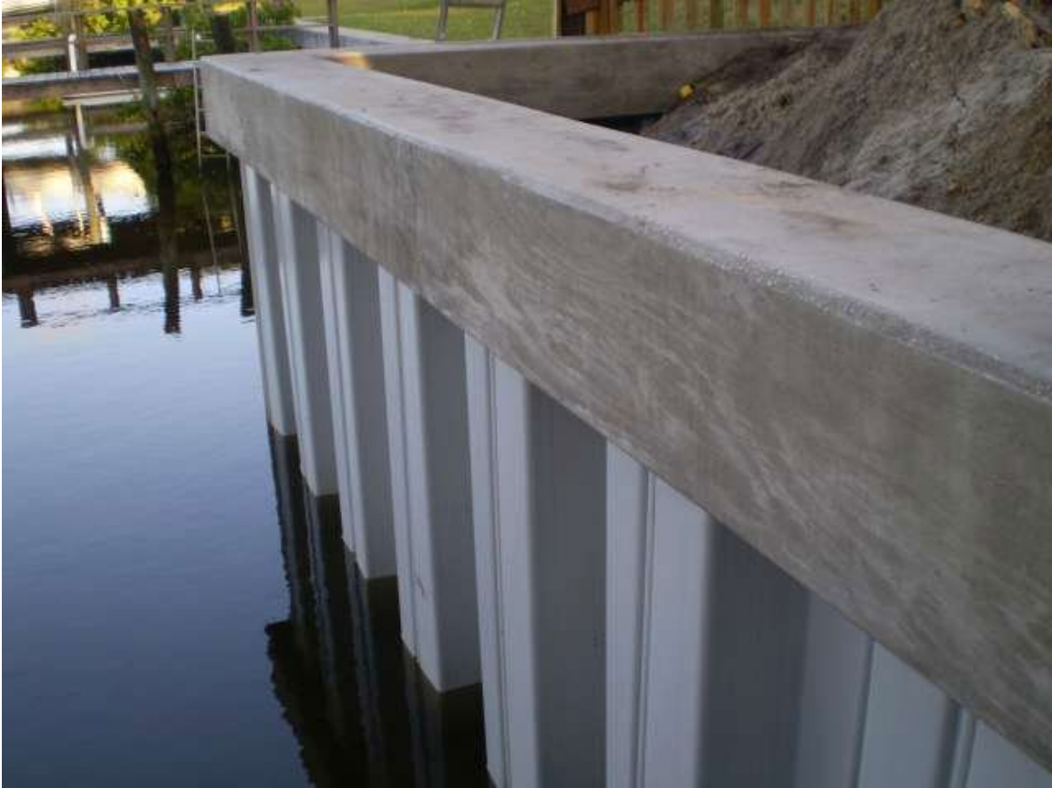
Figure 2-1. Sheetpile Floodwall
